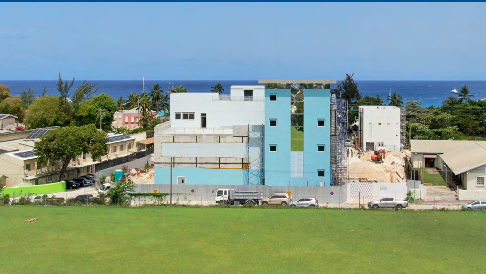
Photo: Bayview Hospital undergoing its updates.
